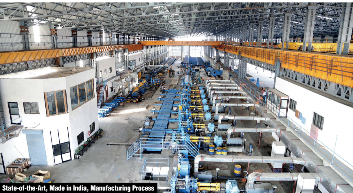
State-of-the-Art, Made in India, Manufacturing Process
